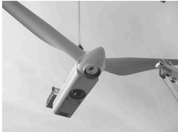
图5-27 Horns ReV风电机组兔耳式安装
